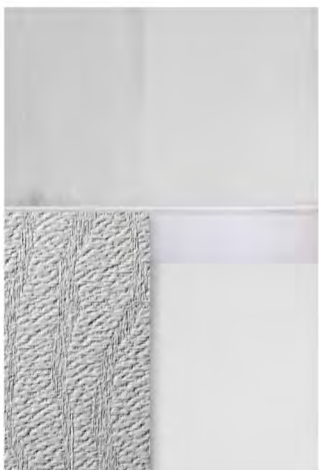
Dry fit transition cap/corner guard placement location and adhere to substrate using contact adhesive
