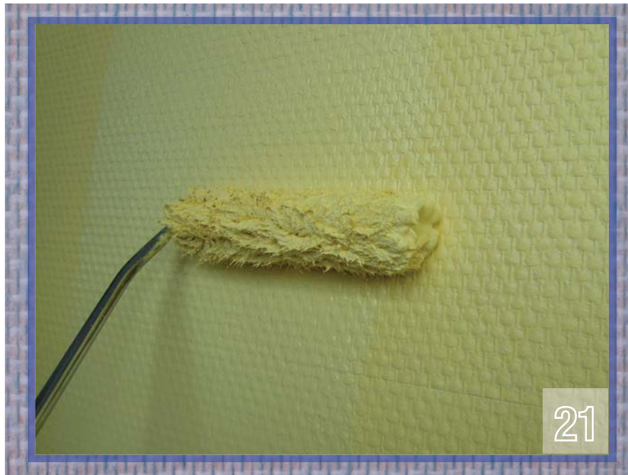
Mending of the transition area (if required, paint wall completely).
