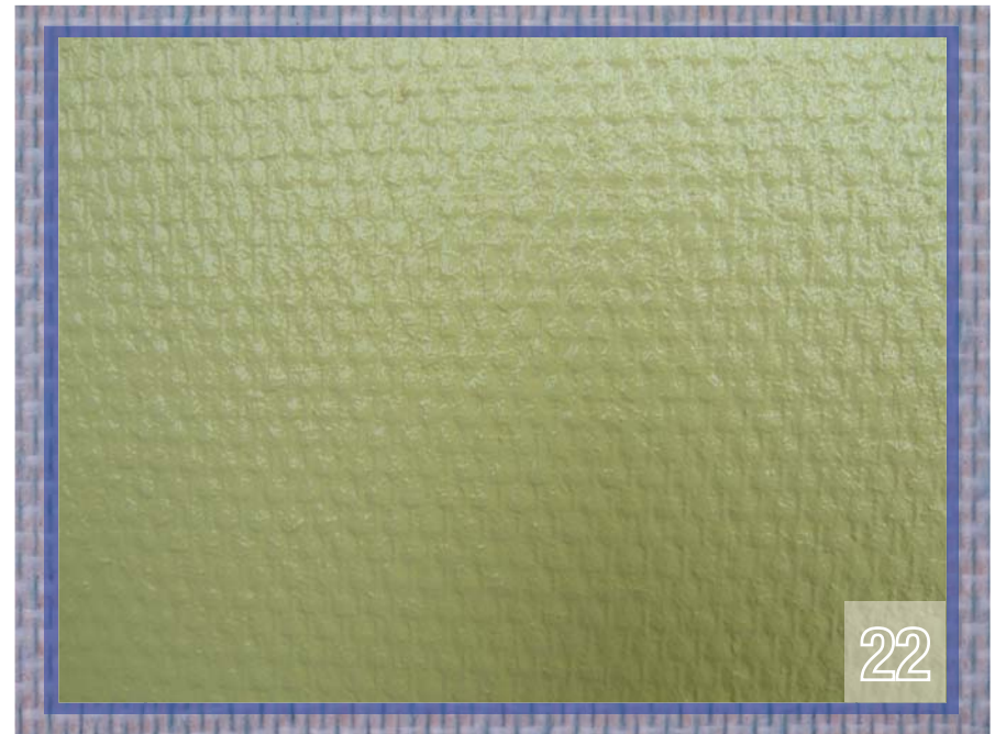
Repaired area after painting.
