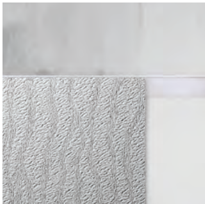
Dry fit transition cap/corner guard placement location and adhere to substrate using contact adhesive
