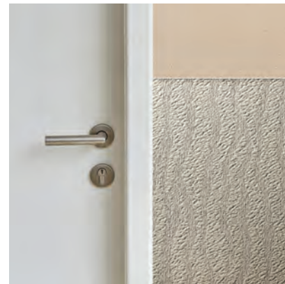
Install Vitrulan base fabric leaving Transition Cap/Corner Guard edge exposed, let dry and finish with specified coating
